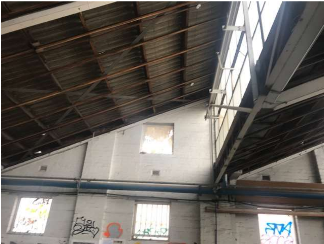
Figure 6 Internal view of saw-tooth roof
