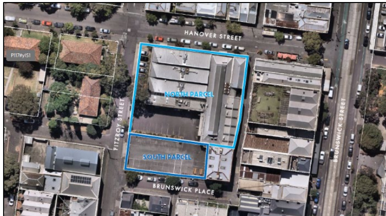
Figure 36 64–66 and 68–70 Hanover Street – aerial
