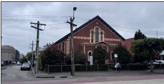
Figure 70 159 Victoria Parade (former Ebenezer Particular Baptist Church) – street view
