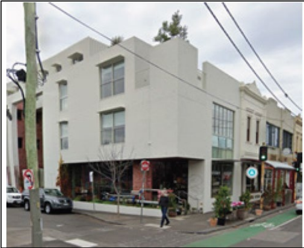
Figure 2 Corner Leicester and Brunswick Streets – 3 storey street wall
