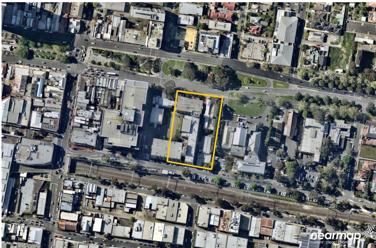
Figure 5: Aerial view of 1000 Whitehorse Road
